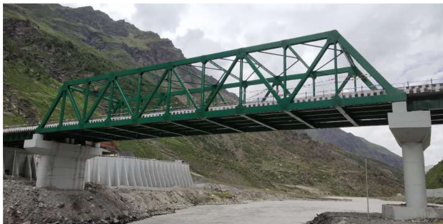
Figure 5.4: Chandra bridge, near Atal tunnel, Teling, Himachal Pradesh, India.
