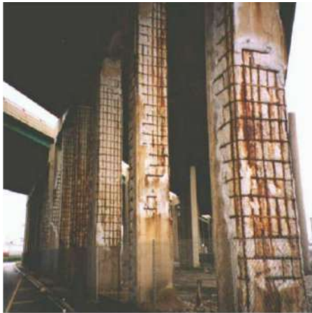
(a) Reinforced concrete steel structure Mohammed (2015).
