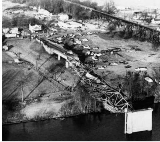
Figure 1.2: Silver bridge collapse due to fracture Matt (2017).
