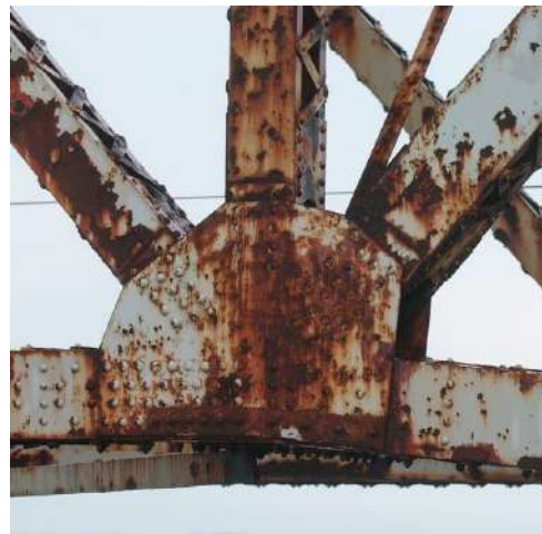
(b) Steel structure Patricia (2014).
