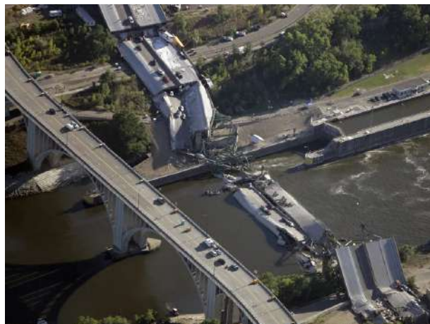
Figure 1.3: I-35 W bridge collapse due to fatigue cracking David (2017).
