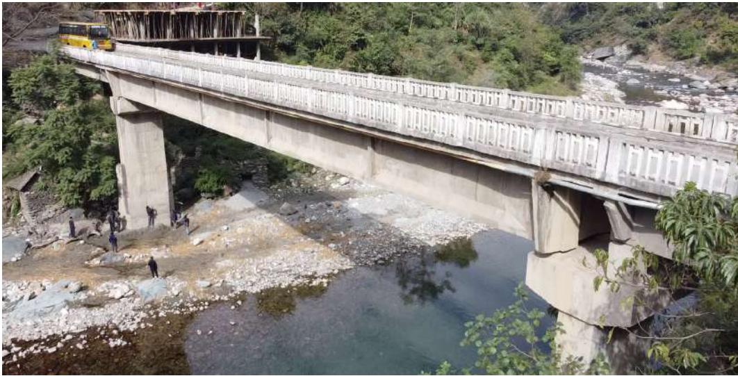
Figure 6.10: Kamand Bridge, Kamand village near Mandi town, Himachal Pradesh, India.
