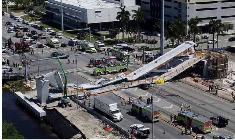
Figure 1.4: FIU pedestrian bridge collapse due to extensive cracking John (2019).
